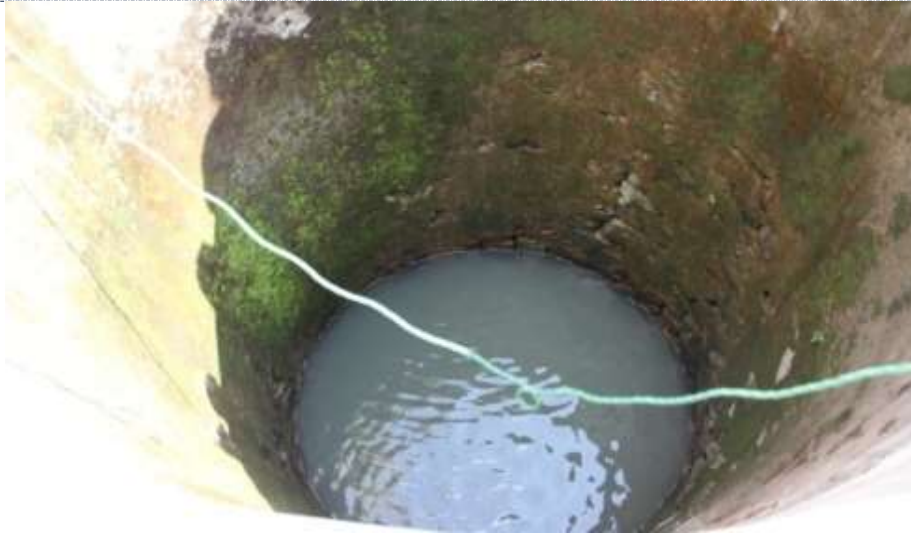
Figures:08 Unprotected open well in Ananthagiri Mandal.
